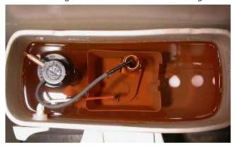
reduce the volume of water used in flushing away waste: varying flush volume, pressure or power assisted flush using a small flush water volume, and reduced flush water volume using a reservoir barrier in th cistern or toilet tank.
