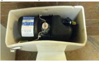
These system traps air and as it fills with water, it uses the water supply line pressure to compress the trapped air inside. The compressed air is what forces the water into the bowl, so instead of the "pulling" or siphon action of a gravity unit, the pressure-assist unit "pushes" waste out
