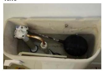
The toilet tank float assembly activates the toilet fill valve as water level in the toilet tank or cistern drops during and at the end of a toilet flush.
