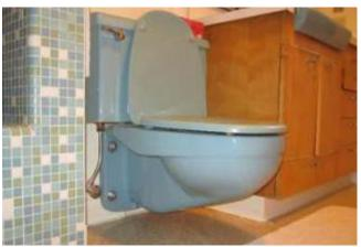
A back-flush toilet that does use a reservoir tank is also produced for special situations such as a location that prohibits installing a drain line in the floor below the toilet. The plumber mounted a back-flush toilet on a short concrete pedestal, raising it just enough to flush into the nearby sewer line found in the wall behind the toilet.
