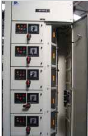
Foam- 4, Type - 7 construction
